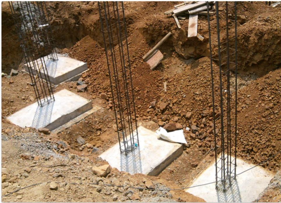
Sapatas isoladas (Fonte: <http://www.understandconstruction.com/types-of-foundations.html>)
